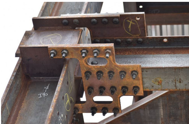
Fig. 3. DuraFuse connection in the MTB2.
