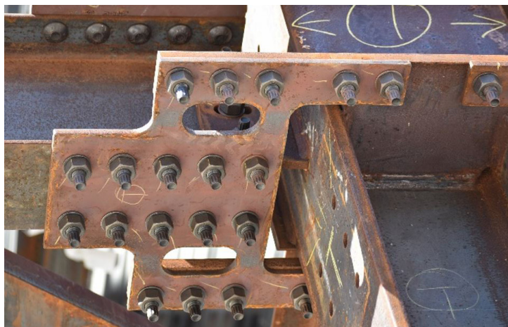
Fig. 5. Fuse plate yielding during severe earthquake shaking.
