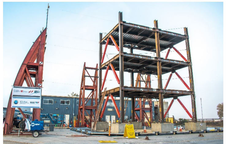
Fig. 1. The upgraded shake table at UCSD with the modular testbed building.
