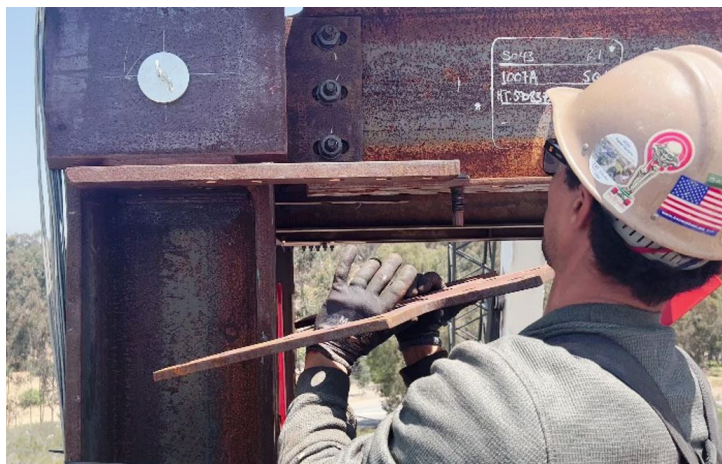
Fig. 6. Fuse plate removal after testing.
