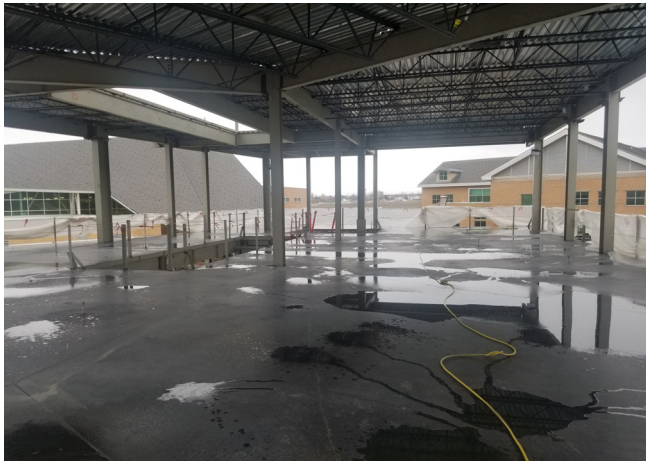
Fig. 3 Level of completion of SLCC Student Center on March 18, 2020 (second floor)
