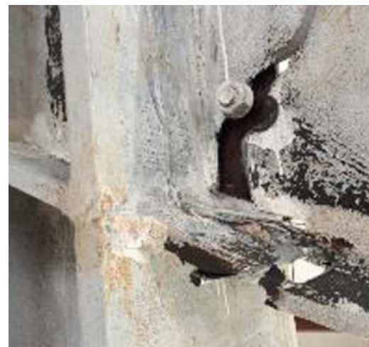
Fig. 2. Ultimate failure observed in sloped connection testing of RBS connections [from Adel and Uang (2019)].
